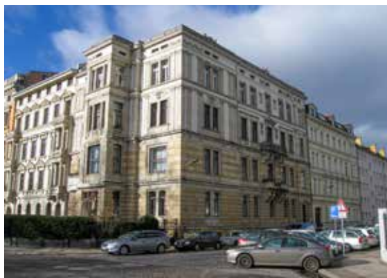
Current view of Hauptmannstrasse 1.
